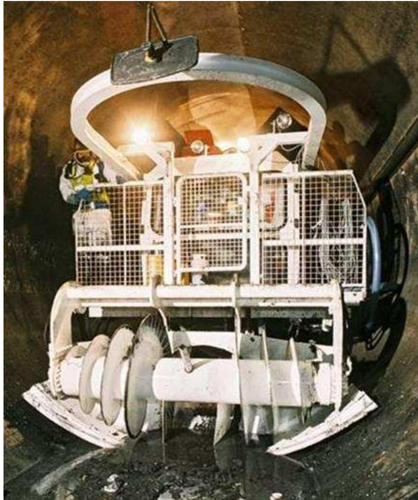
Sewage pipe cleaning system (PROCCOPE)
