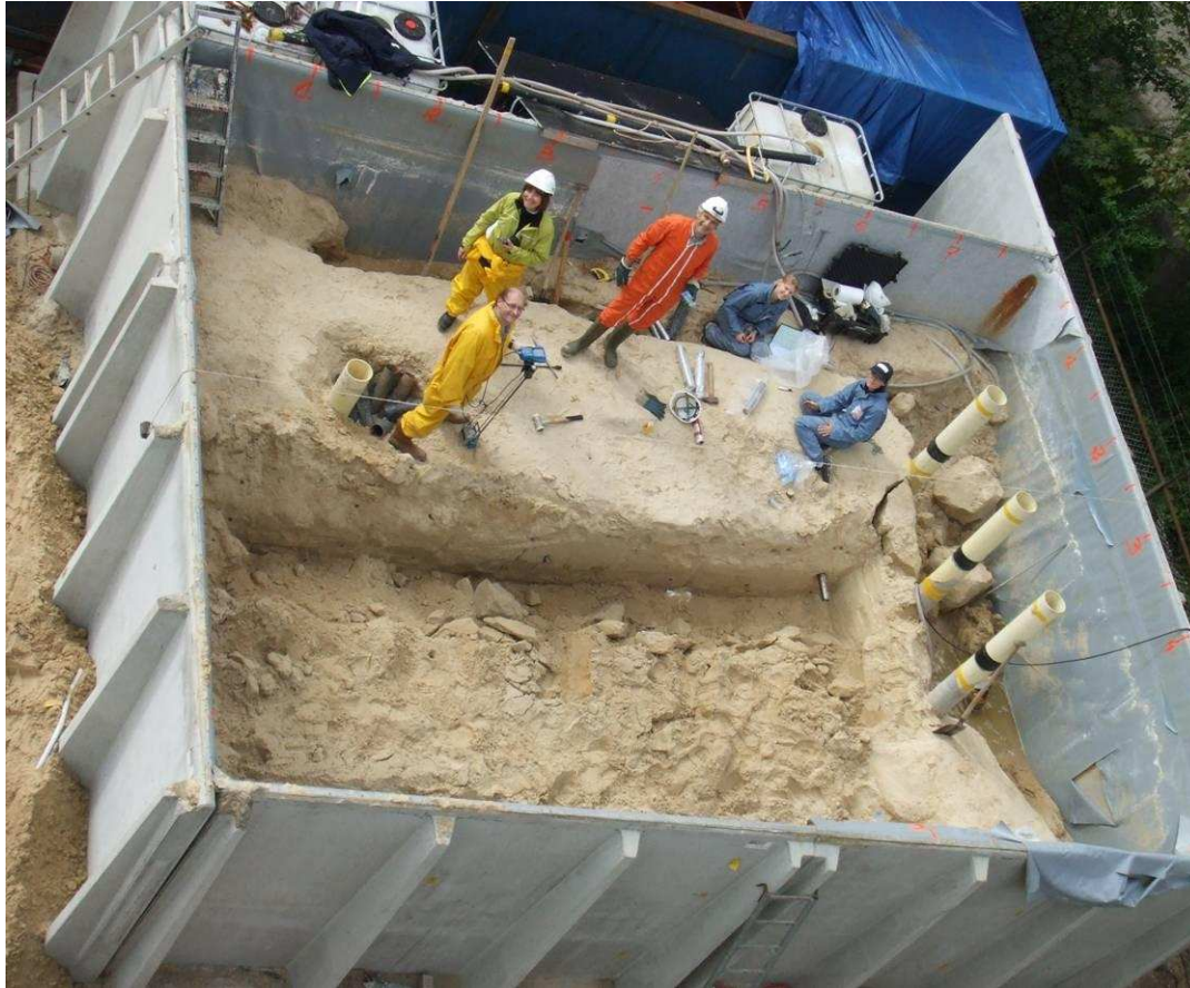
Biocalcis, soil improvement by grouting of calcifying bacteria
