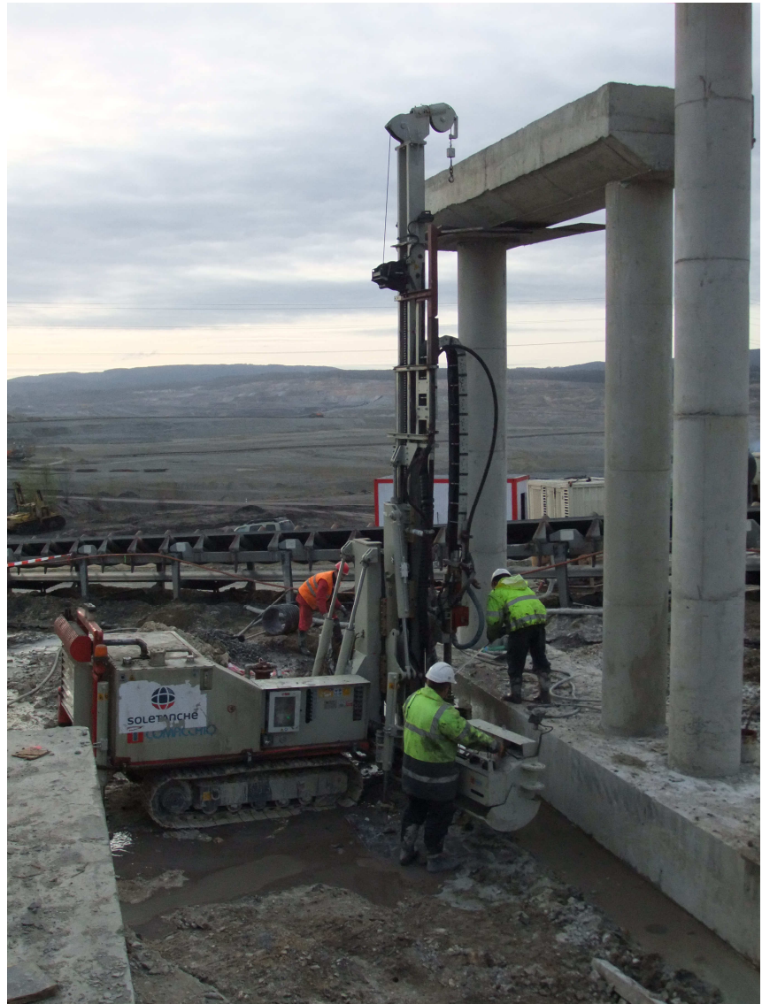
Jet grouting executions under foundations
