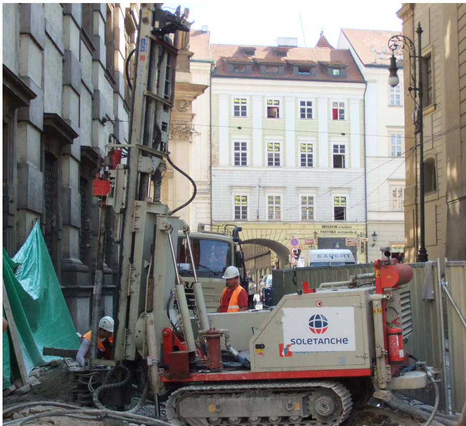
JG works in center of Prague
