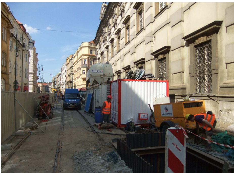
Technology for jet grouting
