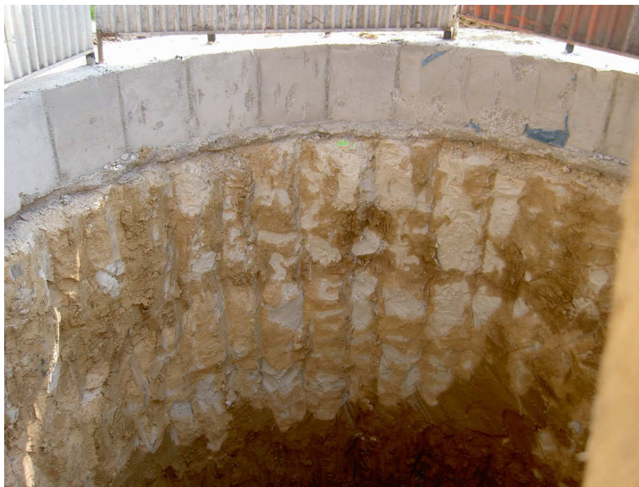
Inner row (JG columns) of circular shaft
