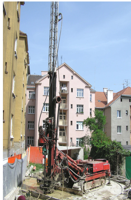
JG works – circular shafts
