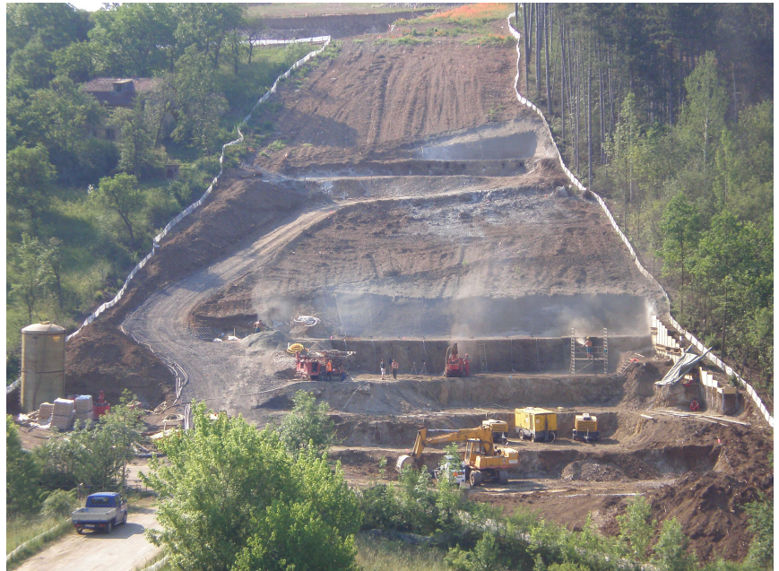
View of jobsite
