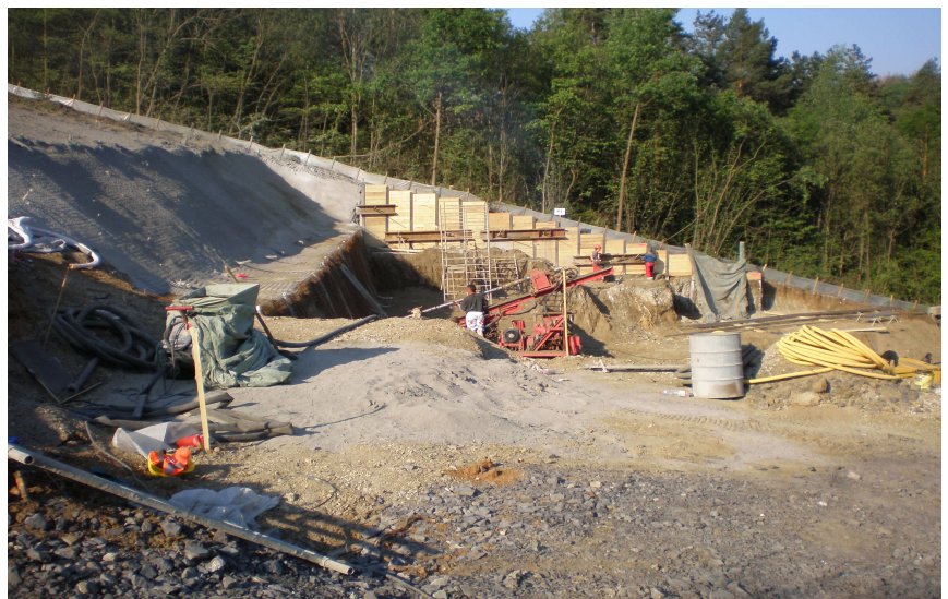
Soil nails realization
