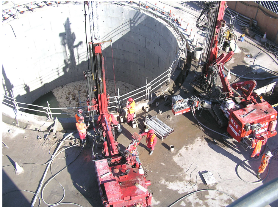
Jet grouting works (Shaft 15)
