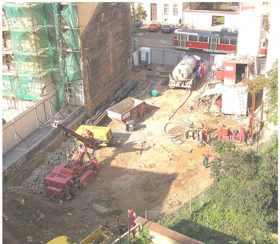
Confined space between existing buildings
