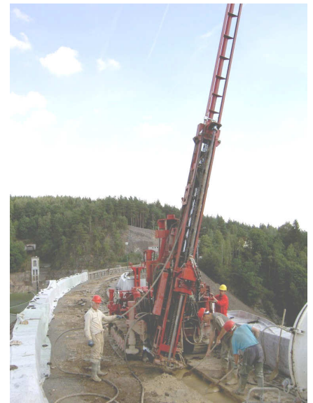
JG works execution
