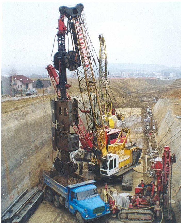
Working on diaphragm wall
