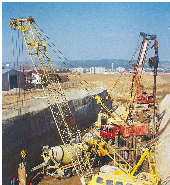
Working on diaphragm wall
