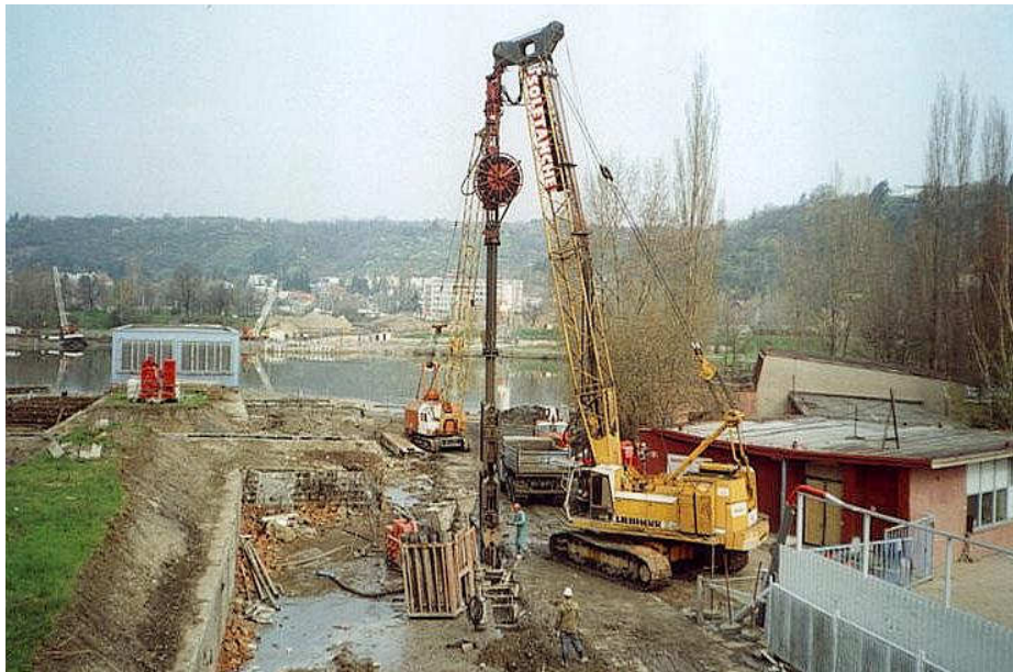
Working on diaphragm wall
