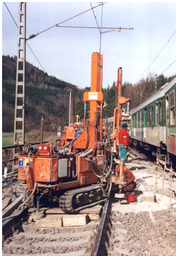
Works next to running trans
