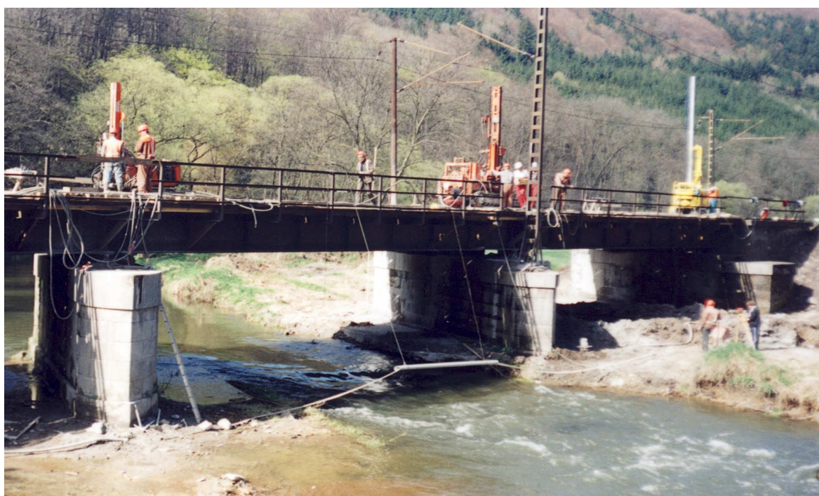
Works on railway bridge
