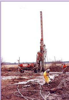
Jet-grouted internal barrier
