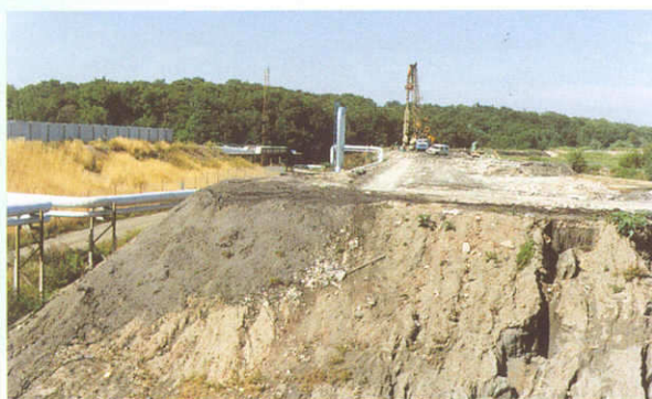
Diaphragm wall under construction from perimeter dyke
