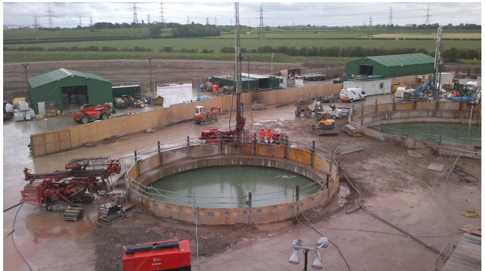
View of shafts S1 and S1A
