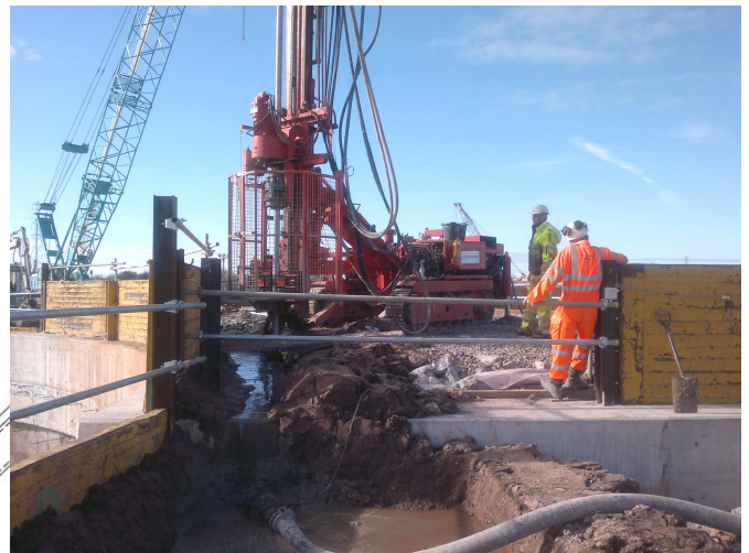
Jet-grouting works
