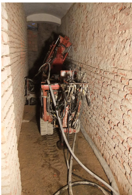
JG works in confined space
