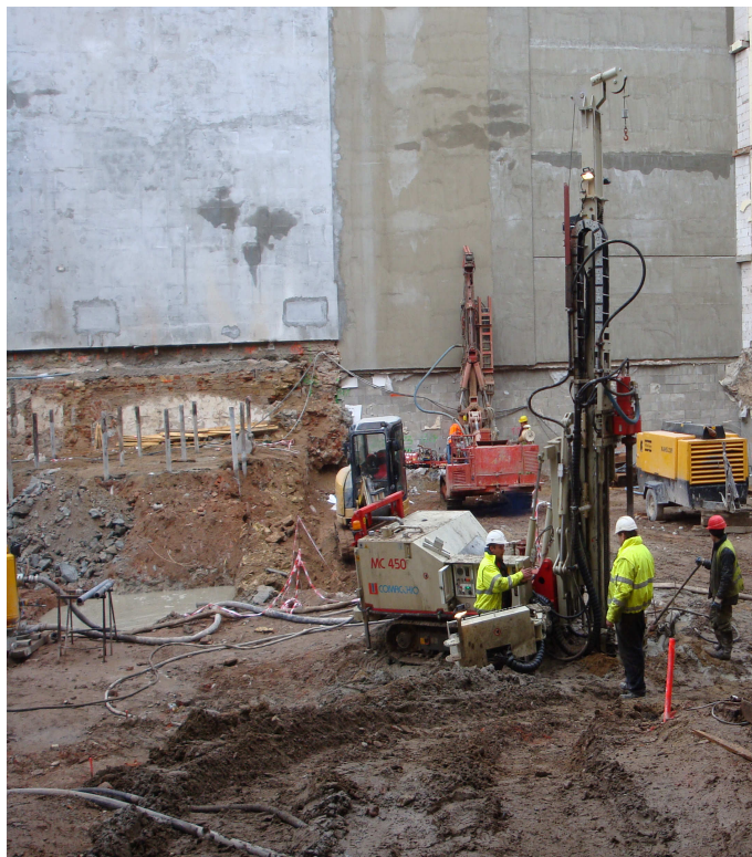
Jet grouting executions – two rigs use
