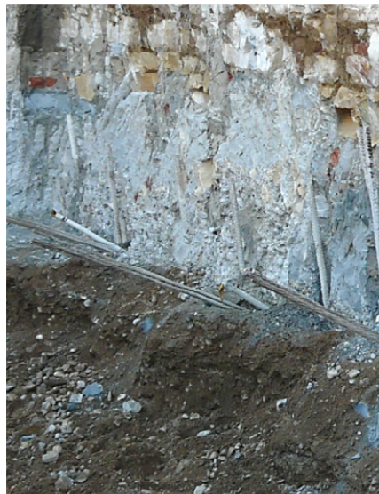
Underpinning by jet-grouting
