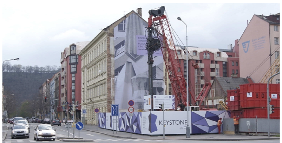
Diaphragm wall executions
