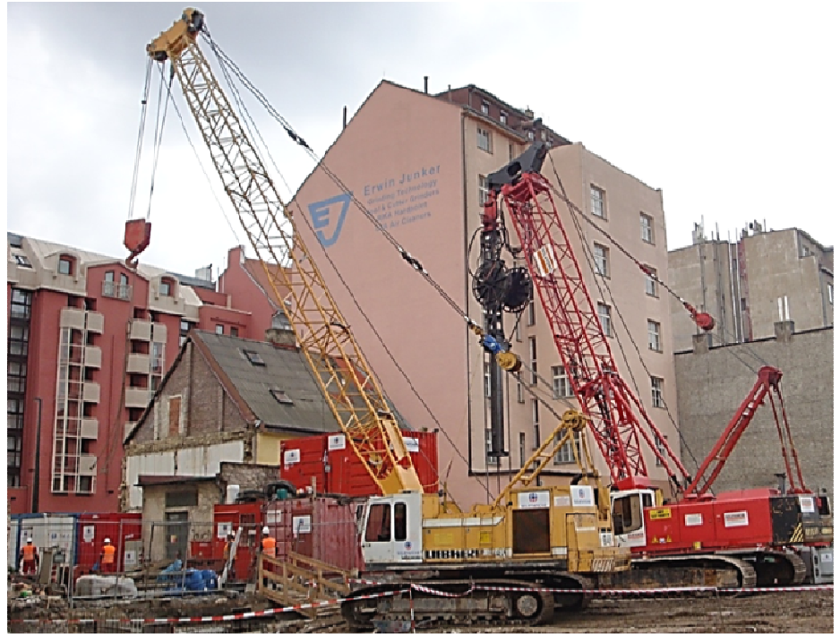
Diaphragm wall executions
