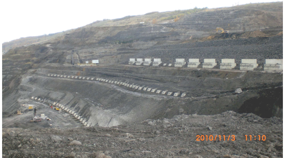
View of anchored permanent block
