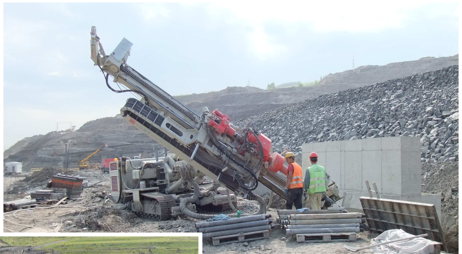
Site works – Anchors executions
