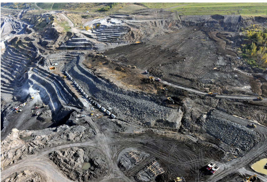
Aerial view of slope secure
