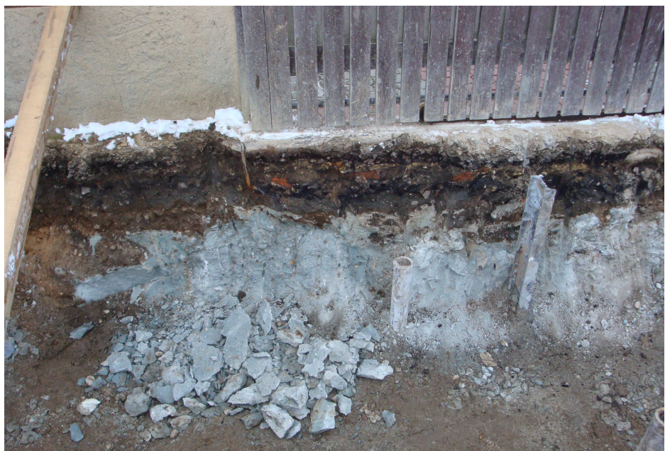
Underpinning of a fence near future anti-flood barrier
