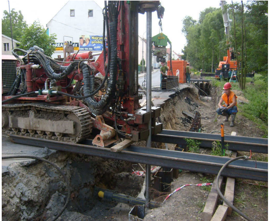
JG works at crossing of barrier and underground services
