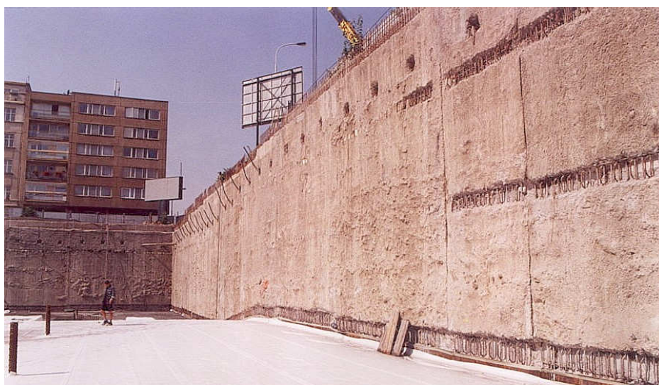
Anchored diaphragm walls
