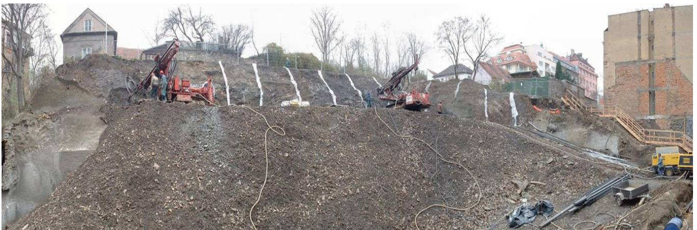
Site works – Anchors and nails drilling
