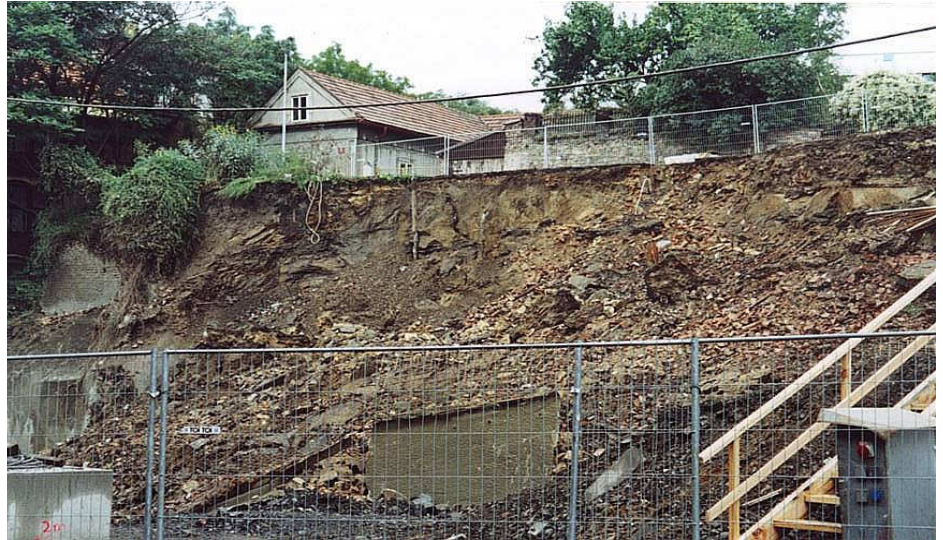
Accidental slope sliding
