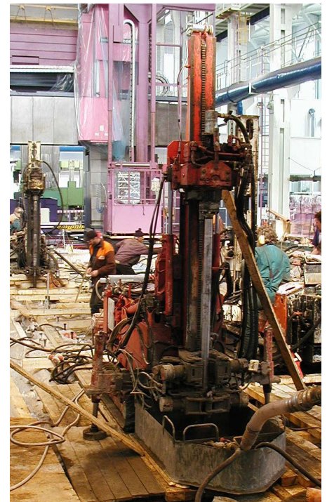
Jet-grouting works
