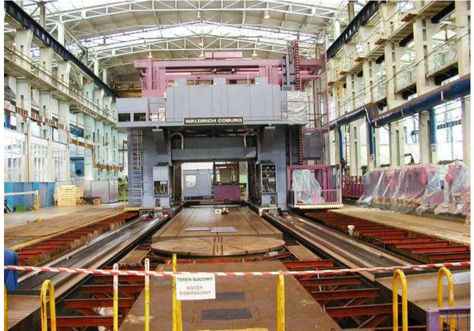
General view of double gantry cutter
