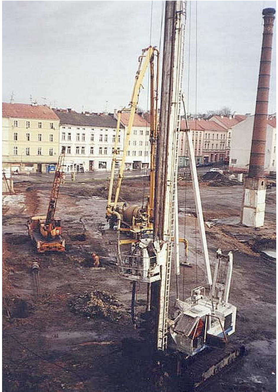
Working on CFA piles
