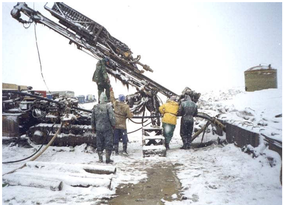
Hard weather conditions – installation of permanent anchor
