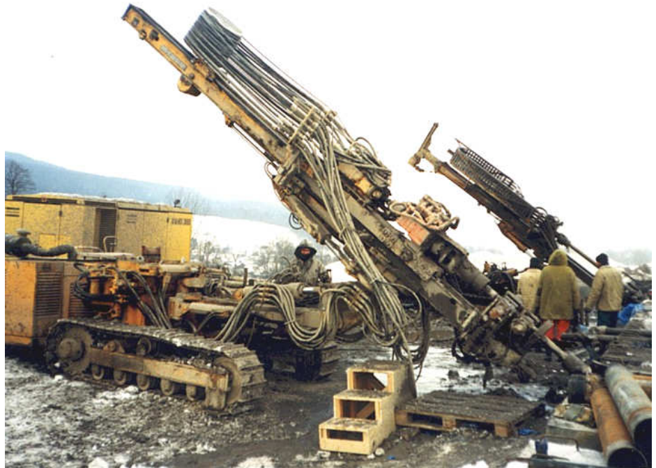
Drilling works for permanent anchors
