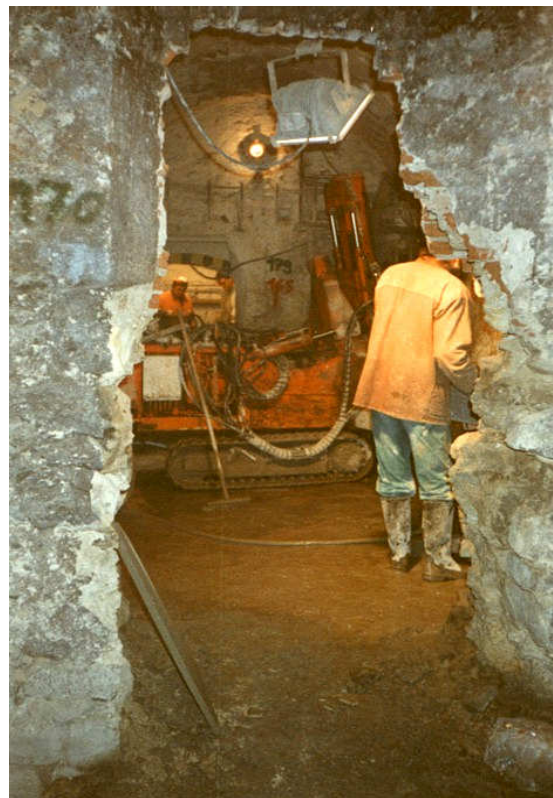
Works in confined space
